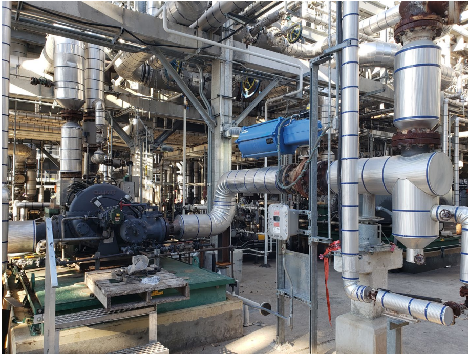
Furnace Charge Pump Turbine Replacement
