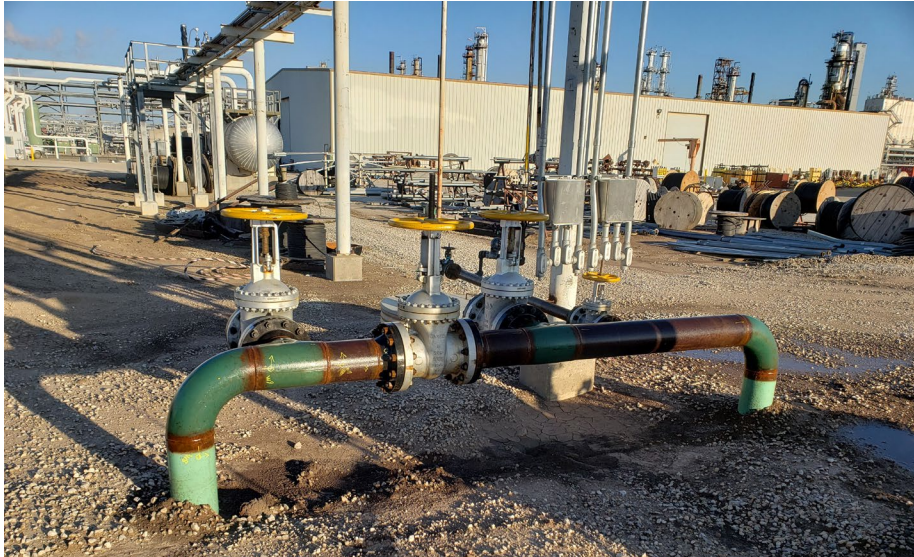
8-inch Natural Gas Line Replacement
