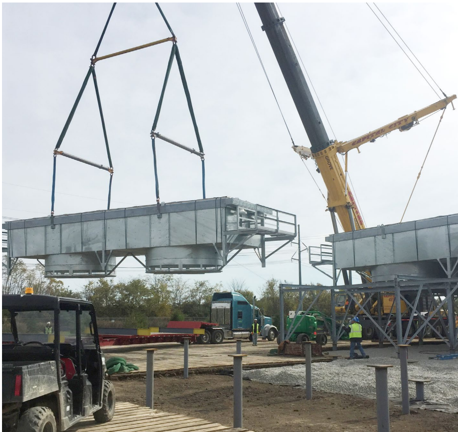
Cooler being installed at Chandlersville
